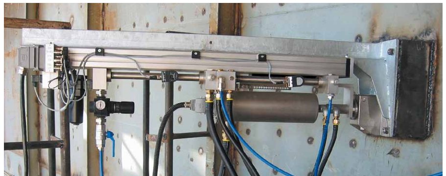
Combustion chamber sensor with retraction unit (water-cooled)
